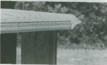
Fig. 18-2. In this view, the top section is lying upside down and a strip of cove molding has been attached to one of the octagonal sides. The ends of the molding are cut at 45-degree angles.
