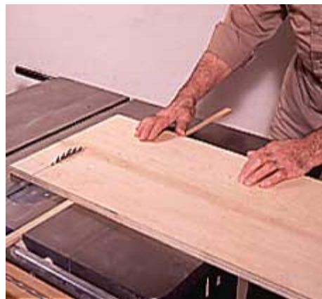
1--Tack nail a strip to the back of each panel. The strip should ride in the miter gauge groove as the panel is being cut.
