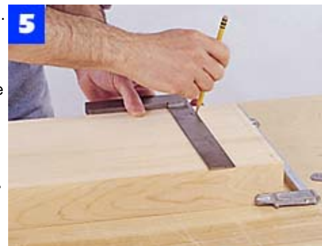
Rip and crosscut the individual bench legs to size, and then clamp them together. Mark out mortise locations on the legs.
