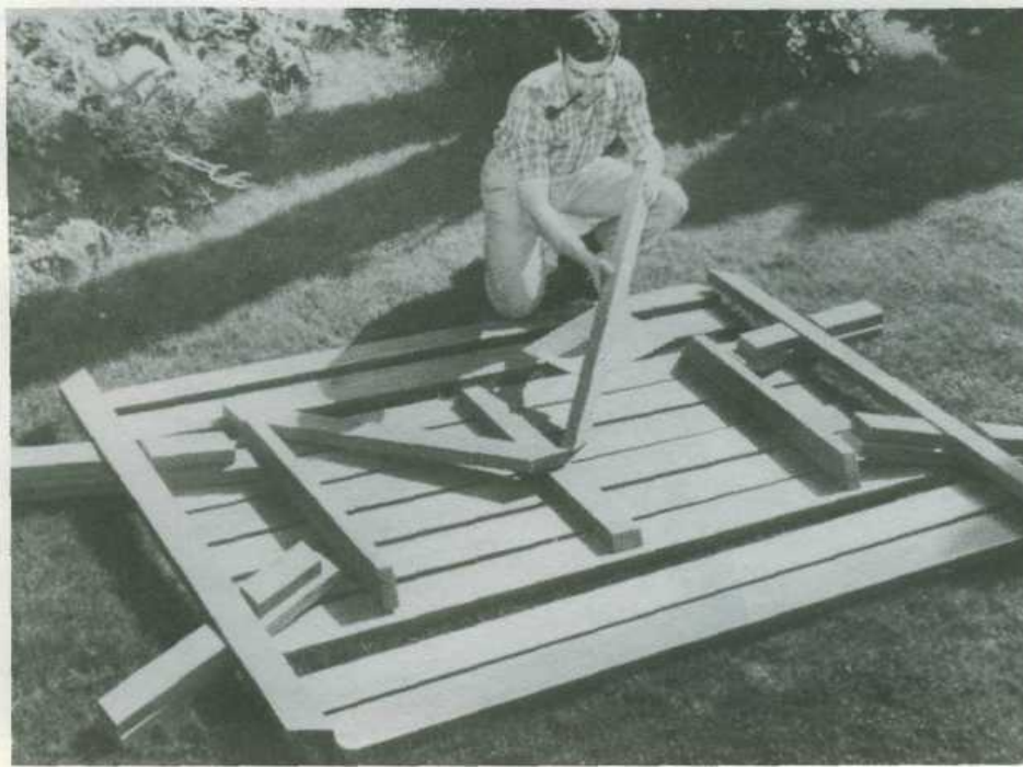
Fig. 14-1. Compact picnic table and bench set accommodates between eight and ten adults. Before beginning actual construction on the set, be sure to lay out all the parts to assure a tight fit.
