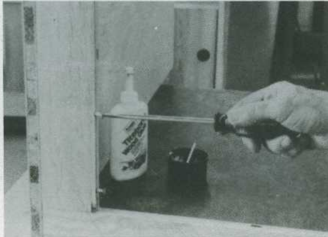
Fig. 24-3. Fasten the top frame to the end panel with glue and wood screws. Exposed plywood edges are banded with wood tape.
