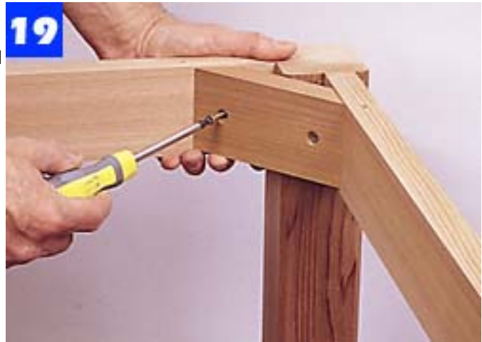
A corner block is installed at each leg on the table and the benches. A pair of screws holds each block to the aprons.
