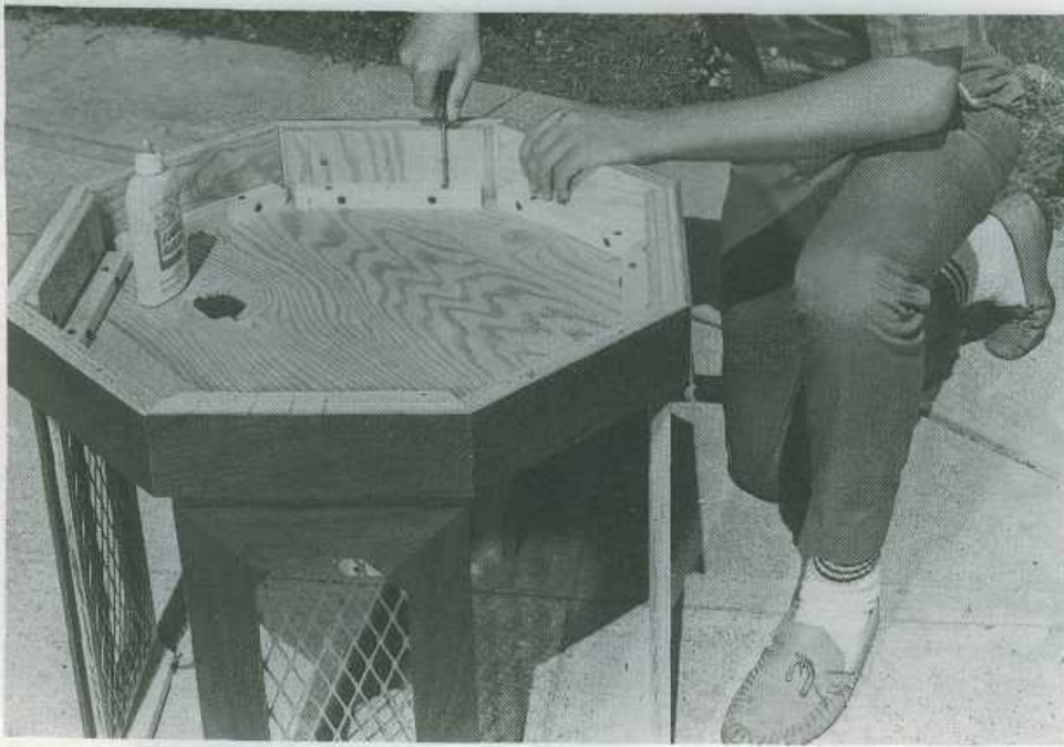
Fig. 18-1. Using cleats throughout the assembly of the unit not only eliminates the need for rabbets and dadoes, but also cuts down on the number of tools required in the construction.
