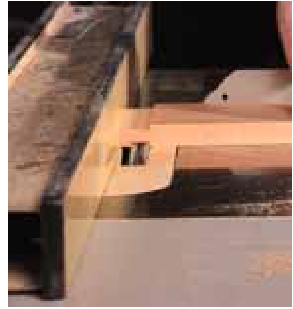
To cut the tenons, use a dado stack on the table saw. Reduce the tenon in thickness by 3/16" on each side.
