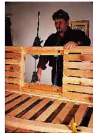
With the notches cut in the support cleats, the two pieces can be glued in place in the seat frame.
