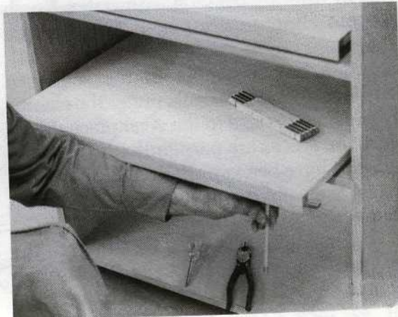
Fig. 1-10. Locating screw holes in VCR platform with pencil. Use awl to make screw pilot hole. Mount door spring hinge.
