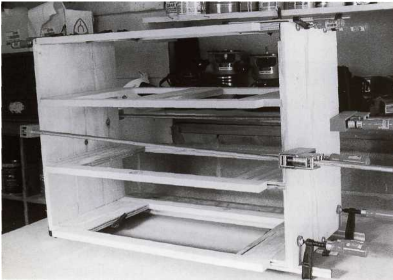
Glue, assemble and clamp the carcass. Note how the front center clamp is set at an angle to pull the structure square.
